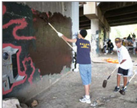
Removing graffiti on the I-70 Overpass.
