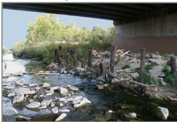
Peoria Street Bridge
