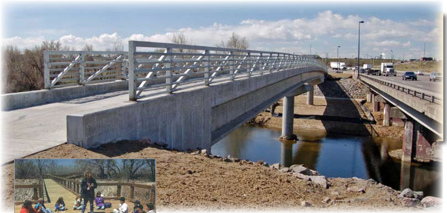
Newly completed overpass and pedestrian bridge on Quebec Street.
